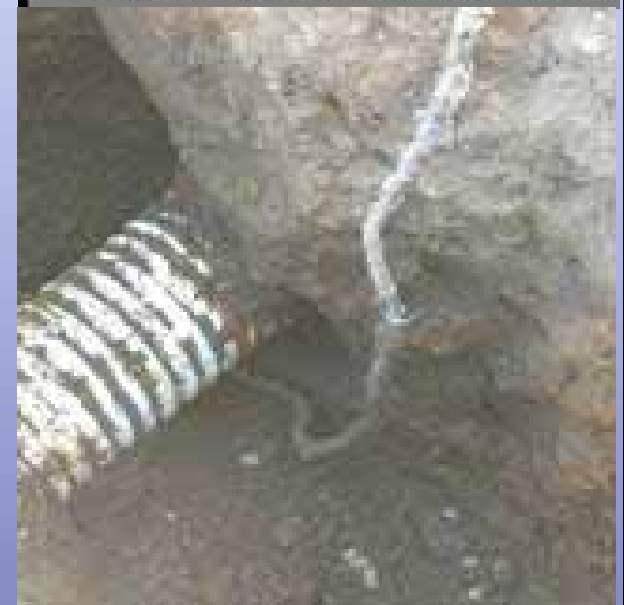
Macropore Connected to Drain (Picture courtesy of Martin Shipitalo)
