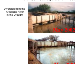
Fort Lyon Storage Canal Headgate
