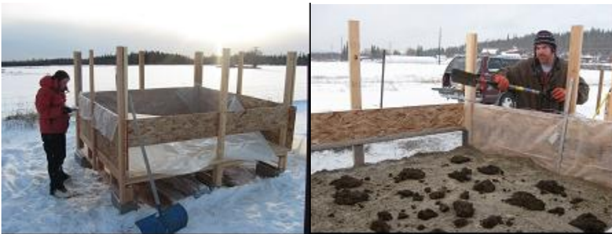
Figure 1: Snowmelt Lysimeter Under Construction (L) and at Startup (R)
